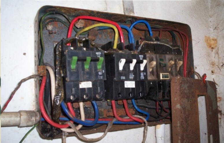
Poor electronic connections
