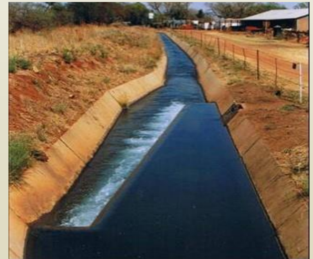
Pressure regulated sluice gate
